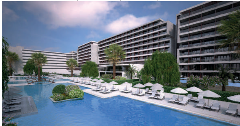
5 AMADA COLOSSOS RESORT, RODHES ISLAND NOVABOND SUPER, NOVACOL FLEX, NOVAGROUT, NOVAGROUT EPOXY
