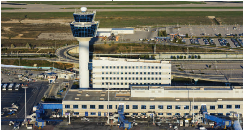
ATHENS INTERNATIONAL AIRPORT MARMOFLEX, NOVAGROUT EPOXY
